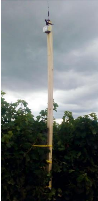
Control unit for soil after installation in the middle of the vineyard
