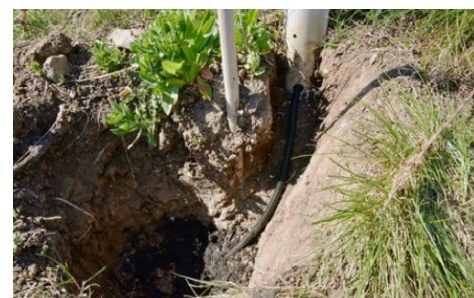
Installation of the soil sensor in the row with fertilizer
